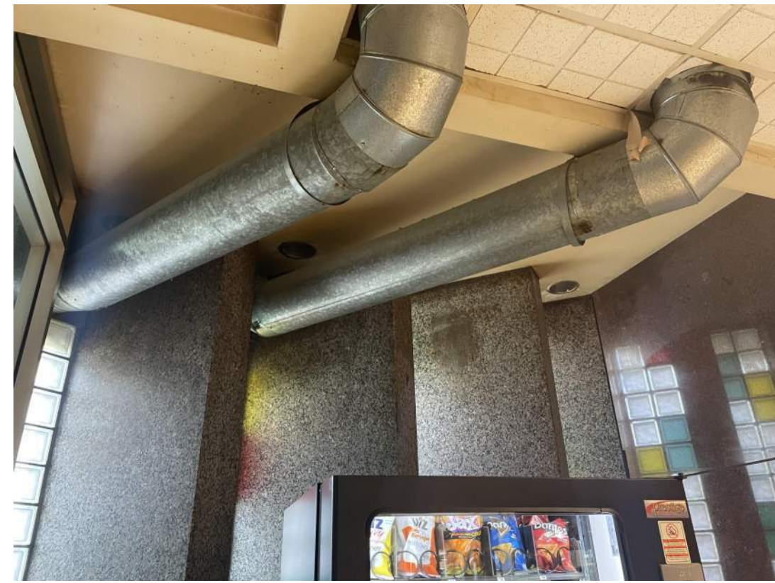
1. REMOVAL OF MECHANICAL DUCTS AND RECESSED LIGHT FIXTURES
