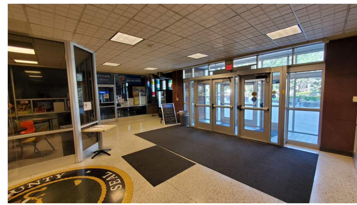
3. REMOVAL OF EXISTING STOREFRONT SYSTEM, REMOVAL OF EXISTING WALK OFF CARPET
